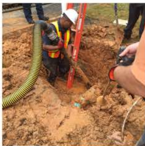
Power Vacs at work (potholing)
